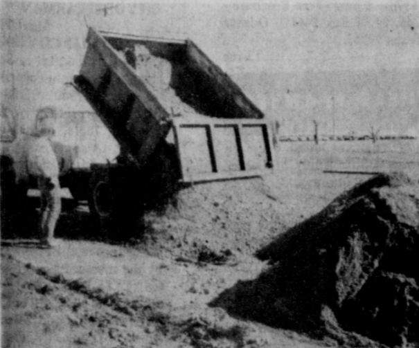
THE NEW PIZZA HUT FOR Spearman is underway! The concrete work will be done this week, and by the last of next week, the top should be going on the new building!
