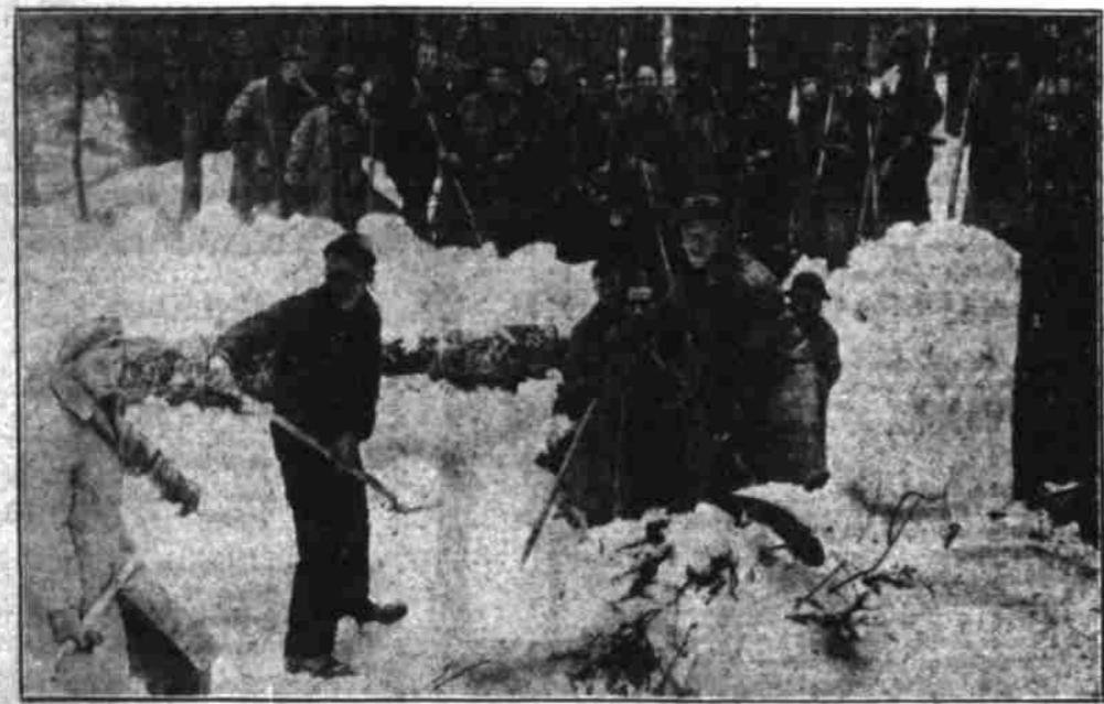
"The sidewalks of New York were never like this, in July," said members of Company 1232, Civilian Conservation Corps, as they piled into four-foot snow to build tent foundations for their camp at Narada Falls, Rainier National park, Washington. Most of them, recruited from New York's tenements, had never seen trees such as grow on Mount Rainier. (Associated Press Photo)
