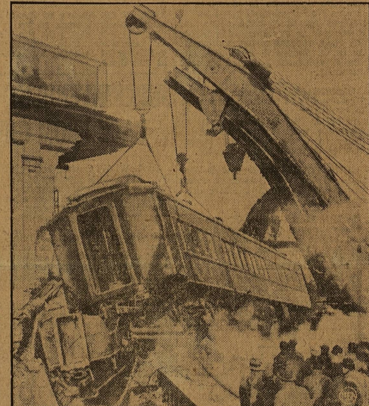
With mighty cranes in action, lifting hundreds weighing many tons, this picture shows the rapid progress being made in clearing the wreckage after the crash of a Pennsylvania railroad train in Pittsburgh which cost at least 10 lives. One of the derailed coaches is being swung upright and another which toppled from the tracks is seen below, with the tender at extreme lower left.
