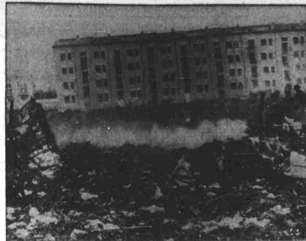
Plane Crash Near Rome Apartment Building
