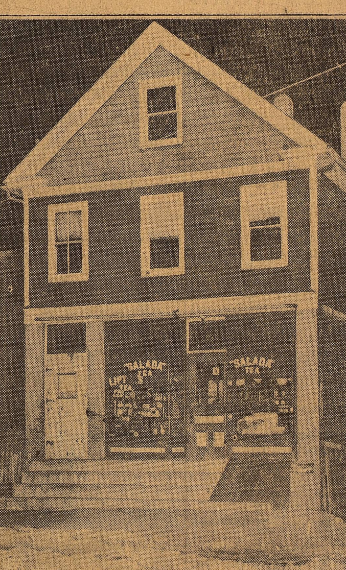
It was in this building—a combination house and store—that Giuseppe Zangara, who attempted to take the life of President-elect Roosevelt, was reported to have lived in Hackensack, N. J. He left here in Sept. 1931, on an automobile trip to the south and last was heard from in Panama several months ago.
