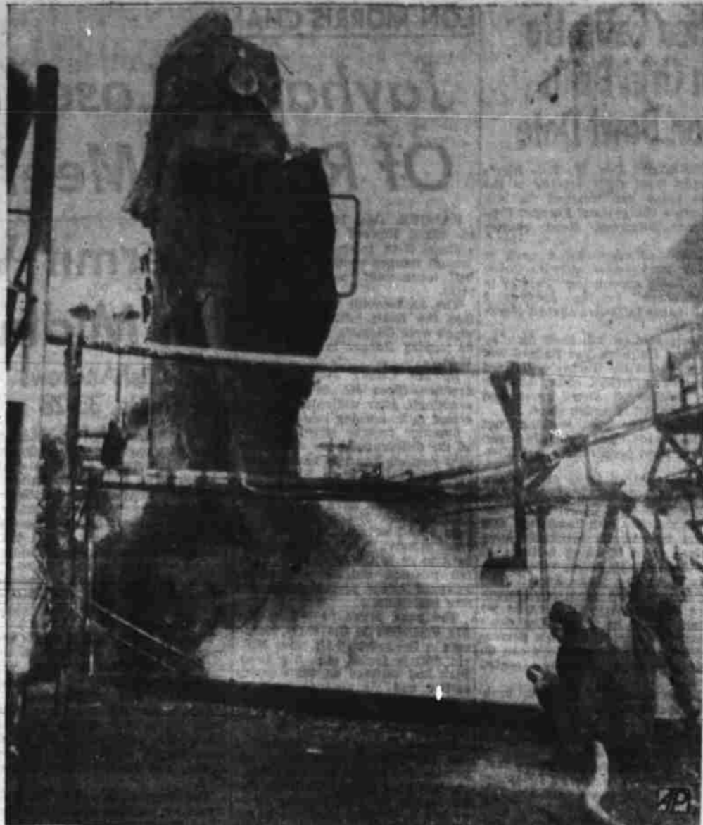
BLAST WRECKS REFINERY TOWER—The big cracking tower (center), a vapor separator, shows a gaping hole after it blew up at the Onyx Oil Refinery, seven miles south of Abilene, Tex. A spectacular fire followed the blast. Firemen at once are playing a stream of water on a leaking gas valve that once connected to the tower to prevent further fire. One man was injured as a result of the blast. (AP Wirephoto).
