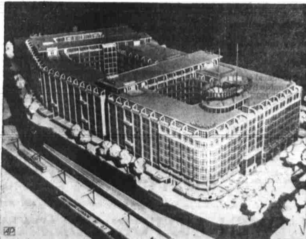
HOLLAND REBUILDS —Model of the new Rotterdam Trade Center, a seven-story building two blocks long, to house organizations which lost their property in the war bombardment.
