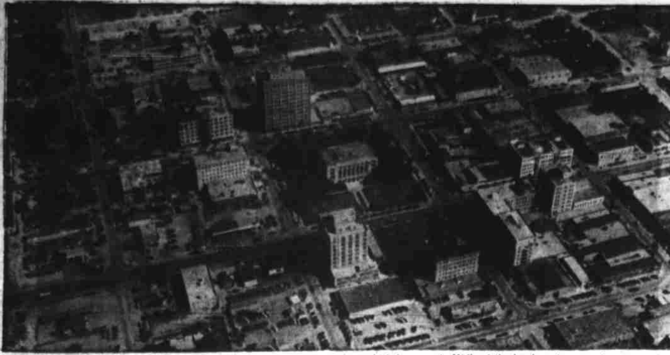
HEADQUARTERS CENTER—Midland, once a placid cattle town which was satisfied with claiming more millionaires per population than any municipality in Texas, today is a city of skyscrapers. Holders of wealth have invested heavily in providing office buildings which have made Midland the headquarters city for a host of oil companies doing business in the area. Midland could still lay solid claim to its millionaire-population boast. Its population today is in excess of 26,000.
