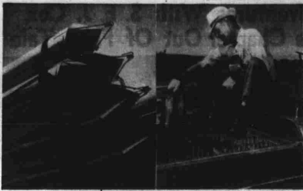
"SOUP" TO OIL—Nitroglycerine, or "soup," as it is called in the trade, has long been an indispensable aid to oil production. This potent explosive is detonated underground to crack hard or "light" oil formations. This expedites flow of oil from the zone. At left are cans of torpedoes. These are filled with "soup" from two gallon cans such as Charles Dublin, veteran "shooter," is lowering into the special rubber lined cases. Sometimes several hundred quarts are used in one shot. Handling the capricious nitro is delicate business. Dublin makes it behave like a kitten. Most people give it a wide berth, but safecrackers have been known to break into nitro stores. (Jack M. Haynes Photo)
