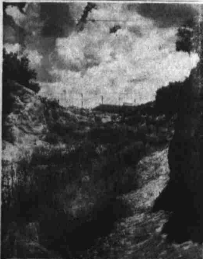
MAN MADE CANYON—A deep canyon, stretching from the baseball park northward to Benton street, marks the locale for the first major development of gravel resources in this area. Most of the gravel put on U. S. 80 and U. S. 87, in the days before first paving came, was scooped out of this canyon. The T&P railroad at one time had a spur into the area as trainloads were shipped to other points. The pit also yielded bones of prehistoric monsters. (Jack M. Haynes Photo)
