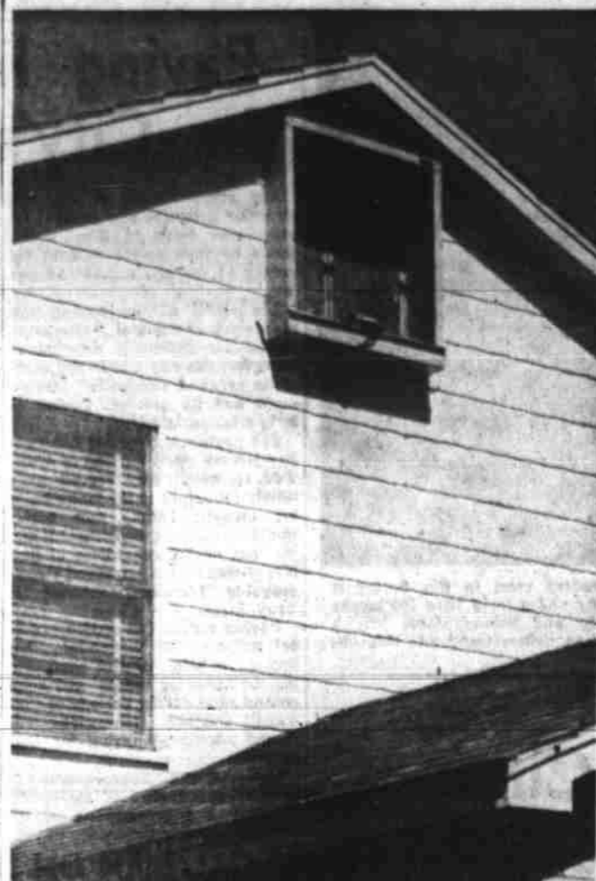
NEW FIXTURE —Of the many transitions in home conveniences, perhaps the newest to find near universal acceptance is that of "air conditioning." Hundreds of Big Spring homes have added evaporative coolers. Most of them are platform affairs, siphoning air through water-soaked excelsior into a window. That they are here to stay in some form or another is evidence by the built-in air conditioner above. It becomes part of the house instead of an eye sore. (Jack M. Haynes Photo)
