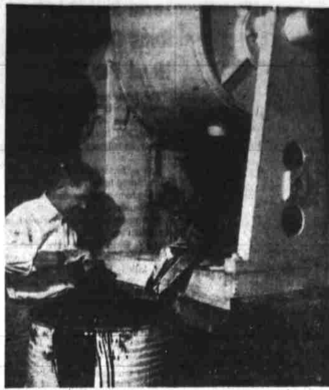
PAINT PRODUCTION —One of the newest manufacturing concerns on the Big Spring scene is the Cactus Paint company now rounding out its first year. Above, Murph Thorp, president, makes a test on the grind of a batch of industrial paint to control its fineness. Products are finding markets from Tulsa, Okla. to the West Coast as well as in this area. (Jack M. Haynes Photo).
