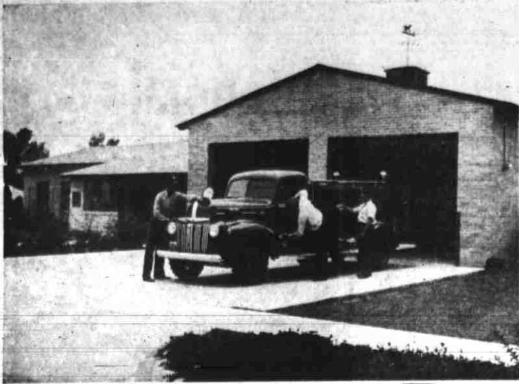
READY TO GO — Firemen at the city's new sub-station at 18th and Main use spare time to keep their red fire truck shined and ready to go, day or night. The station was activated this year, at a cost of more than $30,000. It affords much quicker coverage of the city and relieves demands on the central fire station. (Jack M. Haynes Photo).
