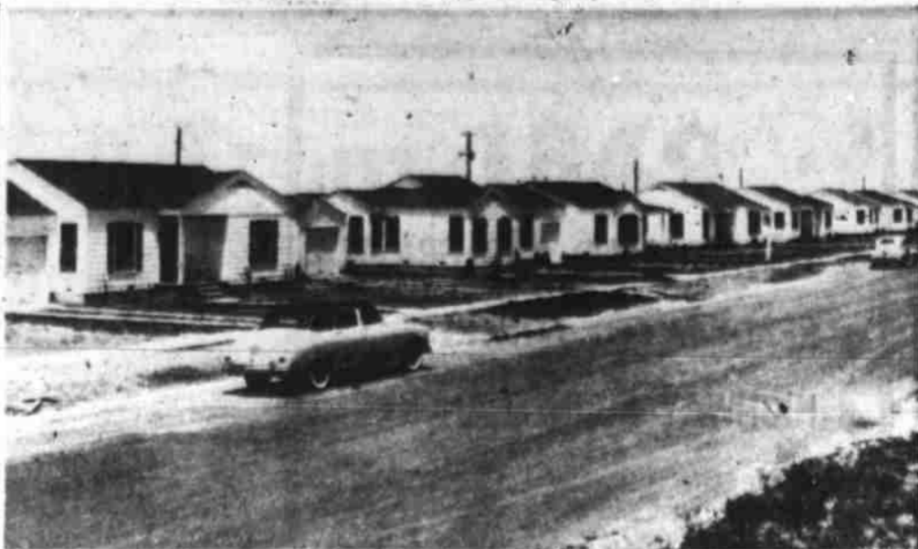
UNIT HOUSING DEVELOPMENT —To meet the mass demands for new housing, several projects have been executed to build up solid areas with new, economical individual home units. Houses above are typical. Largest single project was the Washington Terrace program in 1949. More persistent, however, have been the several unit developments under direction of Louis Thompson, who holds the distinction of having built more homes than any other Big Spring individual in the past decade. (Jack M. Haynes Photo)
