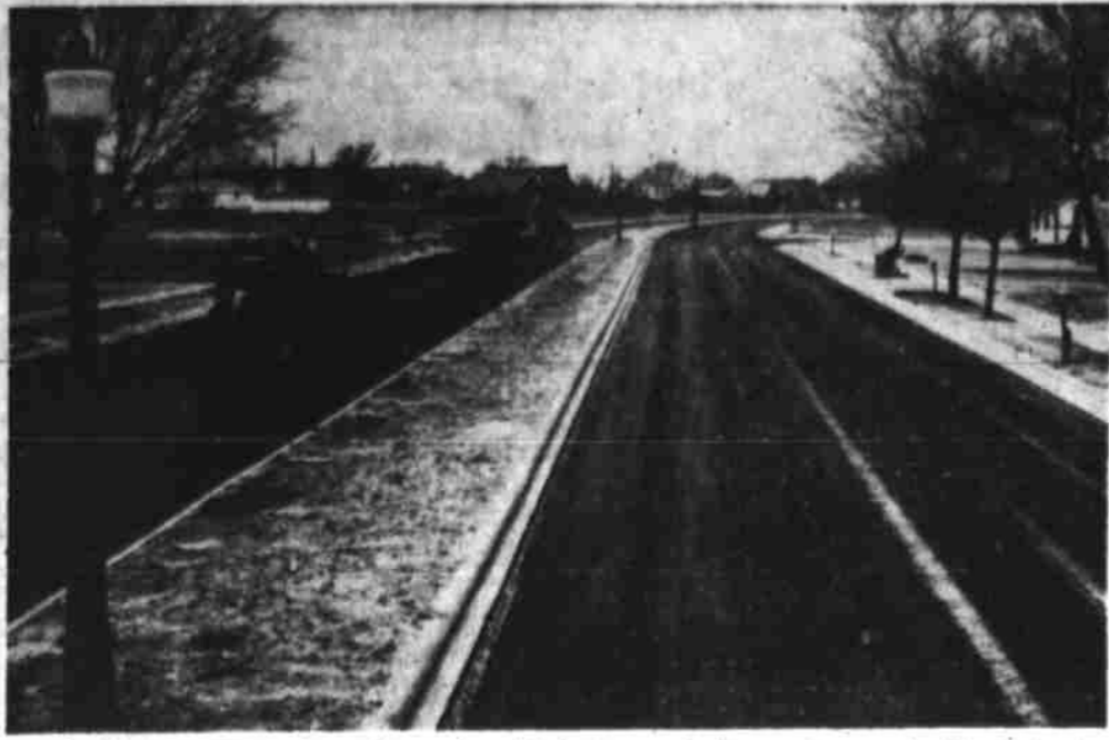
MAJOR IMPROVEMENT —One of the major civic improvements in recent years in Big Spring is that of two large-scale paving projects. In less than two years, the city added more than 200 blocks of new pre-mix asphaltic surfacing. How it transformed a once-dusty, bumpy street into a modern boulevard is shown above. Between three-quarters and a million dollars went into this improvement alone. (Jack M. Haynes Photo)
