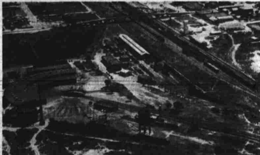
T&P TRANSFORMATION—Half a century has made a tremendous difference in the size and appearance of the Texas & Pacific shops in Big Spring. Above, the early-day shops show the coal chutes to the right, a big cypress water tower in center background and the roundhouse at right. Trees which later became giant cottonwoods were saplings at the time the picture was made. Below, is the million dollar layout opened Oct. 22, 1930. At left is the 23-stall roundhouse with power and boiler plants at front left. Blacksmith and machine shops are behind the roundhouse, the 10-foot turntable in front. In the center is the storehouse, auxiliary buildings and five-car repair shed. A portion of the yards and the Gregg street over-pass are at top. (Bottom Photo by Jack M. Haynes)
