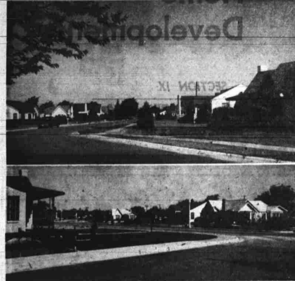
HOMES AND STREETS —Beautification has long been a favorite goal in Big Spring. Within the past decade more progress has been made toward the goal than in all the preceding years. Paving has set up a border from which residents are landscaping and building with pride. Above, a view from Jefferson down Lincoln demonstrates an open, trim neatness. Below, a ranch-type fence along Washington Boulevard is set back to provide a sweeping view. (Jack M. Haynes Photo)
