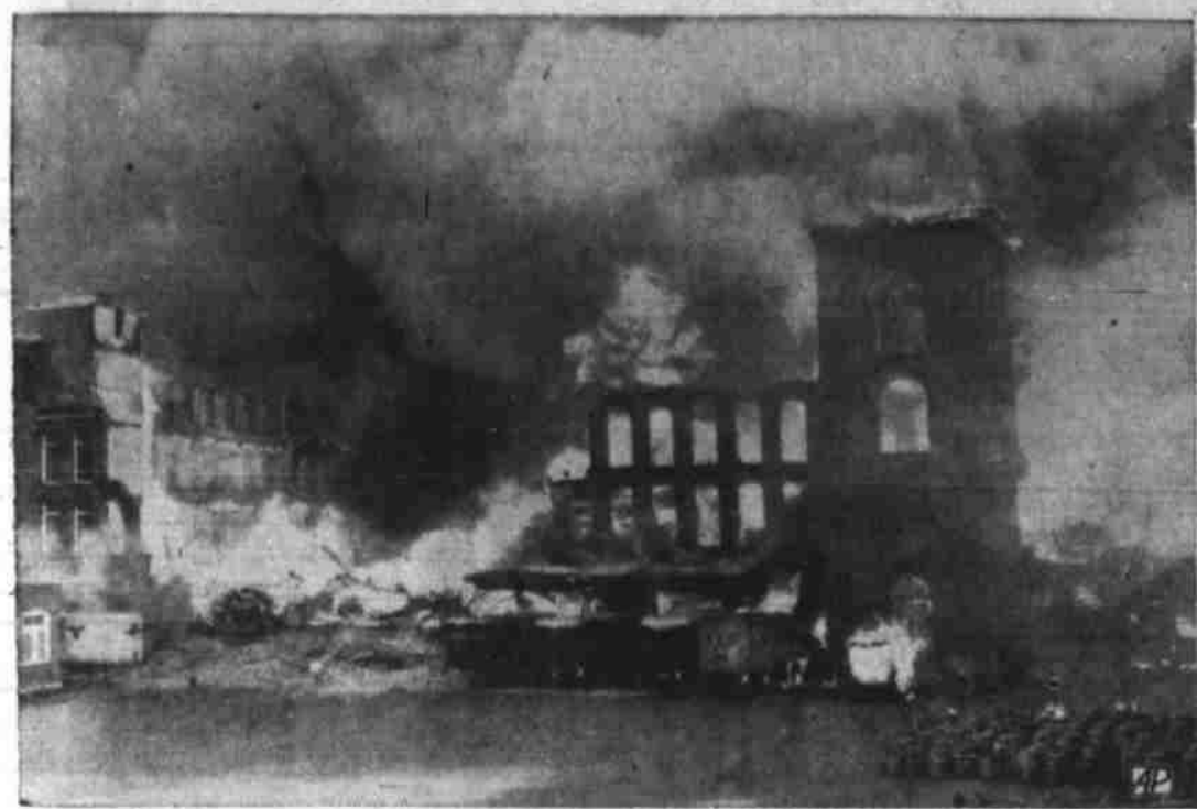
Flames Destroy Mill
