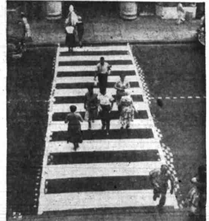
SAFETY DEVICE —Norfolk, Va., traffic engineers provided this crosswalk for pedestrians in the hope that it will prove popular and be seen more readily by motorists.
