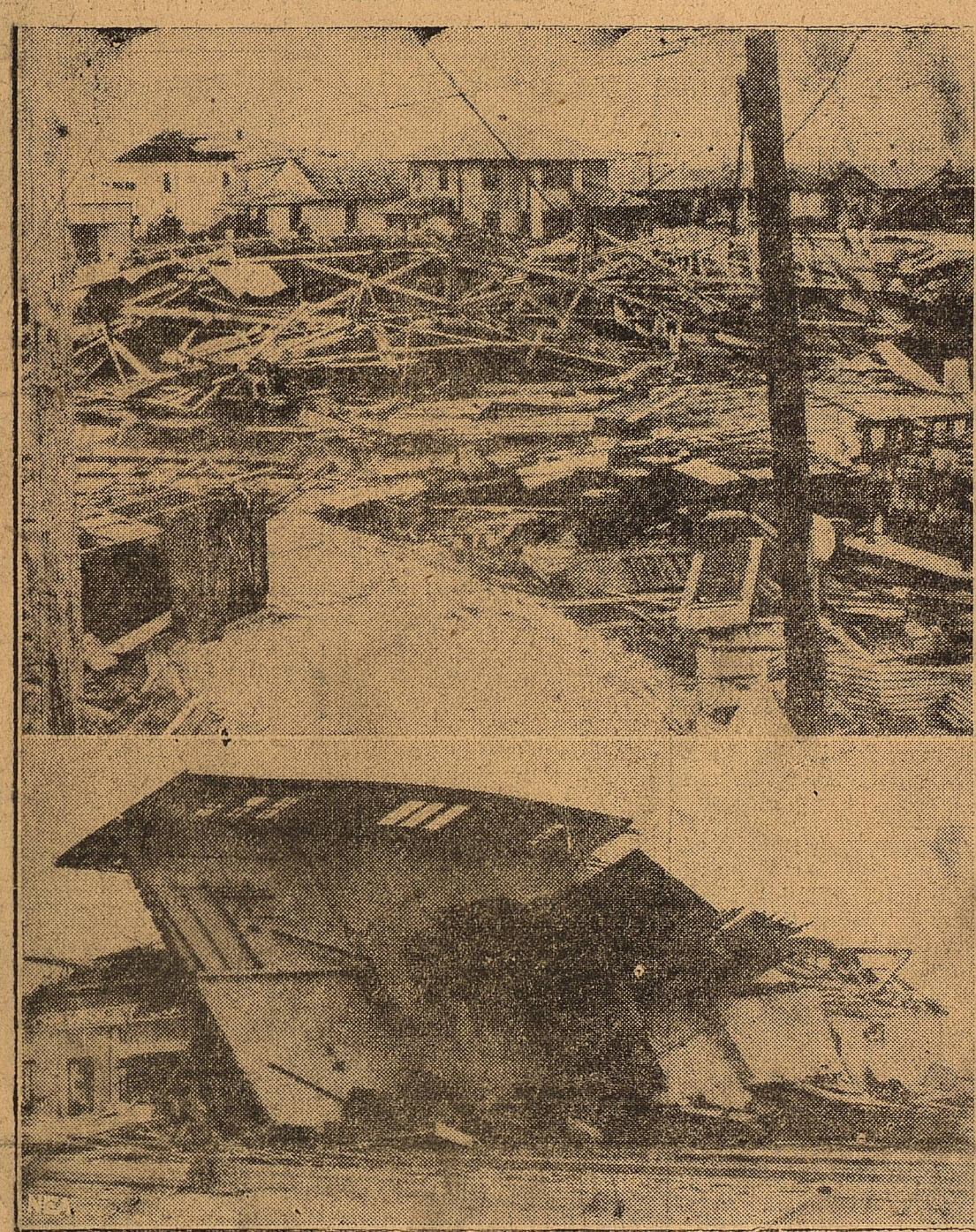
With 35 lives known lost, the hurricane which swept the Texas gulf coast Saturday night left heavy property damage in its wake. Here are two scenes showing the fury of the wind which played havoc around Freeport, Texas. Above, a section of the city showing what happened to the Ford Motor company's plant, and the city's firehall. Below, a lodging house which was dumped on top of the Chevrolet Motor company.
