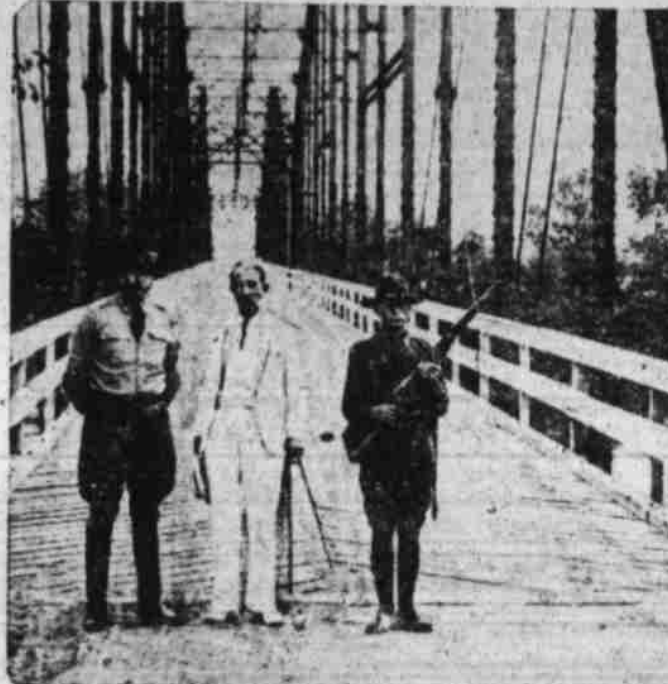
Gov. W. H. Murray of Oklahoma is shown with guardsmen at the Red river toll bridge between Denison, Tex., and Durant, Okla. When a free bridge paralleling the toll bridge was opened, Murray ordered guards to relax their vigilance at the toll bridge. Previously he had ordered an injunction to open the toll bridge approach.
