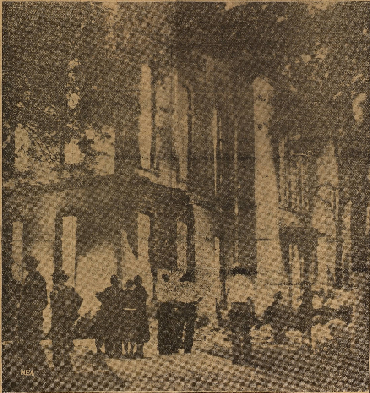
The picture shows the courthouse at Sherman, Texas, as it burned and suffocated a negro in one of its vaults. The mob, a part of whose members are seen fired the building. Immediately after the mob had penetrated the building, the negro was taken out and hanged and dragged behind a car, for one of the most vindictive outbreaks against law and order to have been staged in Texas in months.
