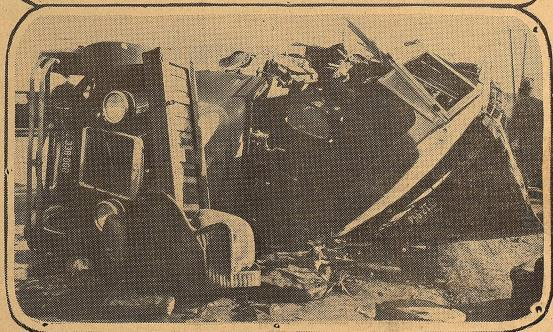
Notice the condition of the All-Steel Top on the Studebaker in the upper picture. This car, after a terrific impact with the bus shown below, rolled over several times and came to a stop more than 150 feet from the point of collision . . . and the Top held its own. A top of weaker
