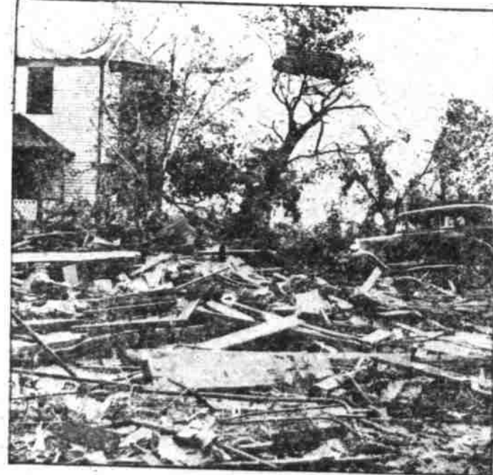
Above is a scene typical of the destruction spread by a cyclone which swept through Eureka, Mo., injuring three persons. The roof was lifted off the house at the left and the auto tossed on top of the wreckage of its garage. Part of a tin roof is wrapped about the tree in center.
