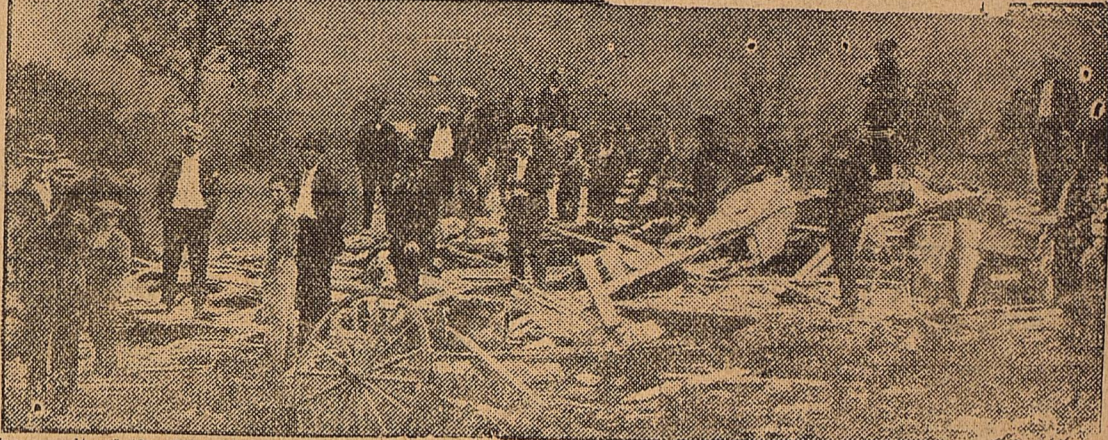
The result of the latest violence in the textile strike area is pictured here. Near Elizabethton, Tenn., the home of Mack Elliott, union striker and former mechanic at the Gantzoff mills, was completely wrecked since the walkout occurred. Elliott and his family had left the house before it was destroyed. Fellow strikers and police are shown examining the wreckage.
