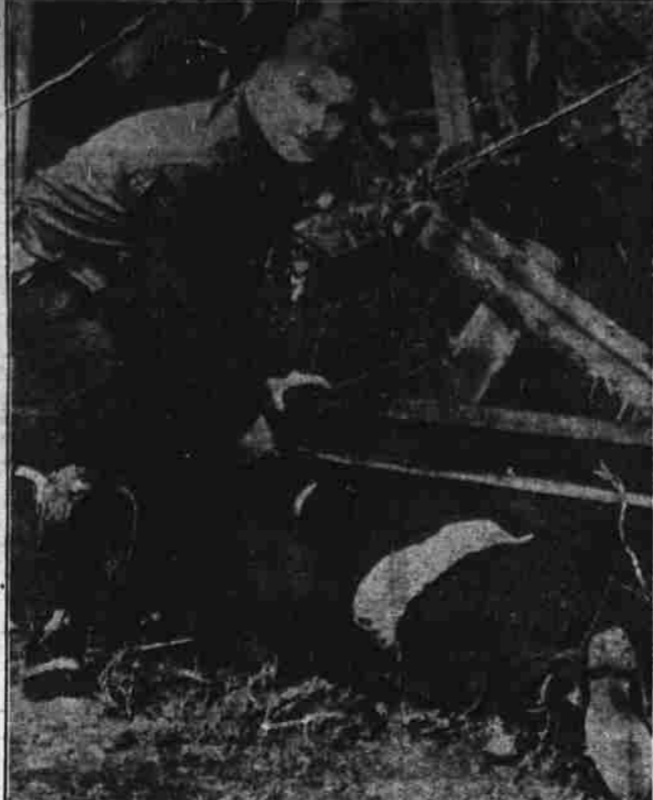
A Los Angeles policeman had a job on his hands when he attempted to extricate this man, one of several persons injured by debris from a night club which collapsed as a result of the southern California deluge and flood. (Associated Press Photo)
