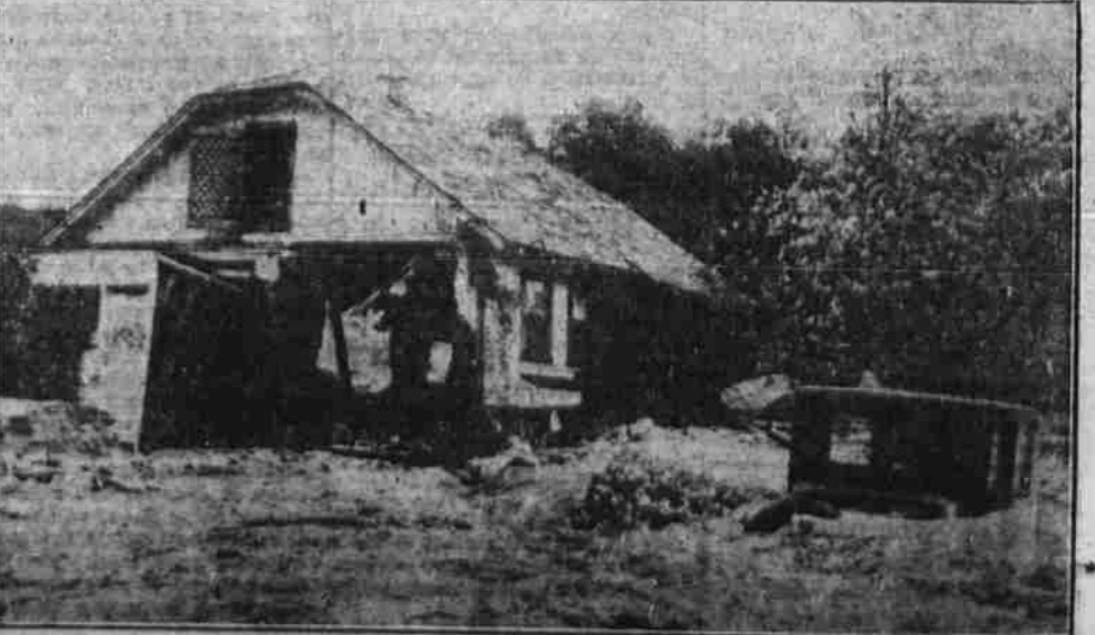
This Associated Press picture, taken near Glendale, Cal., shows how muddy waters of the California flood half-buried homes and cars under silt and debris. This was a typical scene in the heavily damaged foothills area near Los Angeles.
