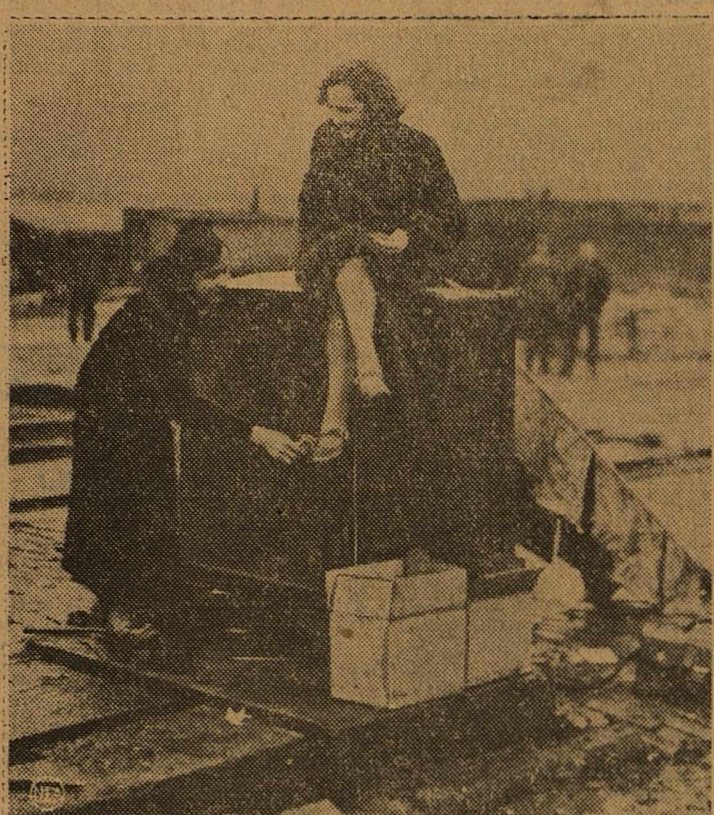
Only sign that a Pittsburg coal company's office ever stood on this site is the safe, on which Mary Hagola, an employe, is working the combination as her sister Anna sits atop the strong-box. There was a good reason for all this interest in the safe, as it contained more than $4,000.
