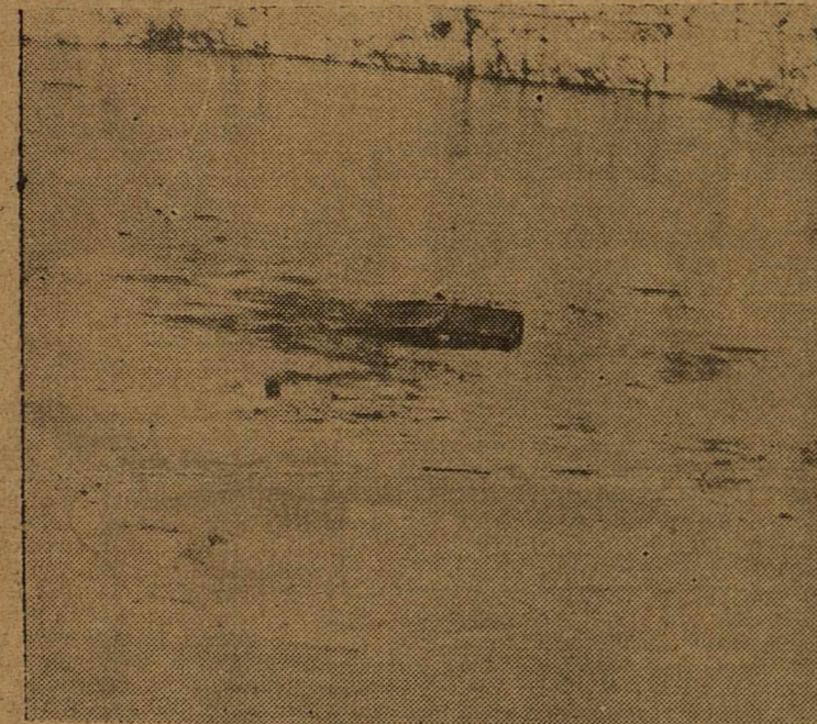
Tragic evidence of the devastation wrought by the flood roaring down the Ohio river is given in this picture, of a shattered house floating down the swollen stream. Its roof barely visible in the tossing waters, it is seen as it passed Steubenville, O.
