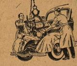
At less cost than an ld-fashioned overhaul, you can exchange your present Ford engine for a factory-reconditioned cylinder assembly. Many other units are also included in this service.
