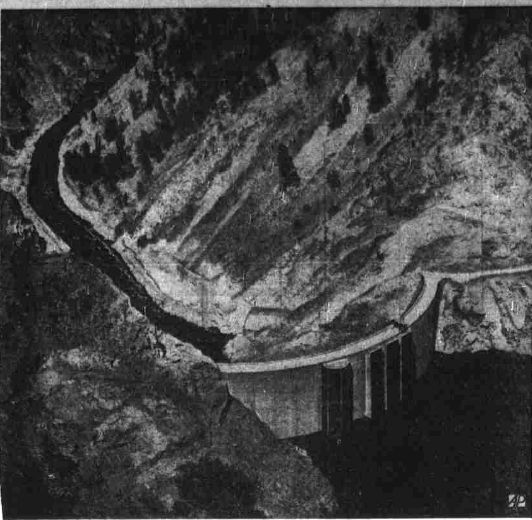
UNCLE SAM DAMS ANOTHER RIVER—Wedged between the steep walls of Seminoe canyon, above 296-foot Seminoe dam blocks the North Platte river and will store 1,020,000 acre-feet of water for the fertile arid lands of Kendrick federal irrigation project, in Wyoming.
