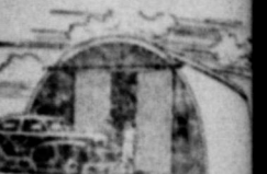
QUONSET 32—32 feet wide; length variable in 10 foot sections.
