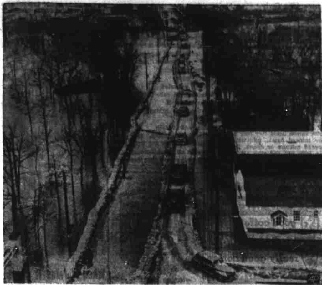
THE ROAD TO ST. VITAL—This ramp is built over flooded-out Marion St., the main road from Winnipeg, Canada, to St. Vital. The bridge (top center) was washed out when the Red River of the North backed up the Seine end flooded this whole area, leaving St. Boniface a virtual island. Normally, the Seine is a very small creek at this point. (AP Wirephoto.)
