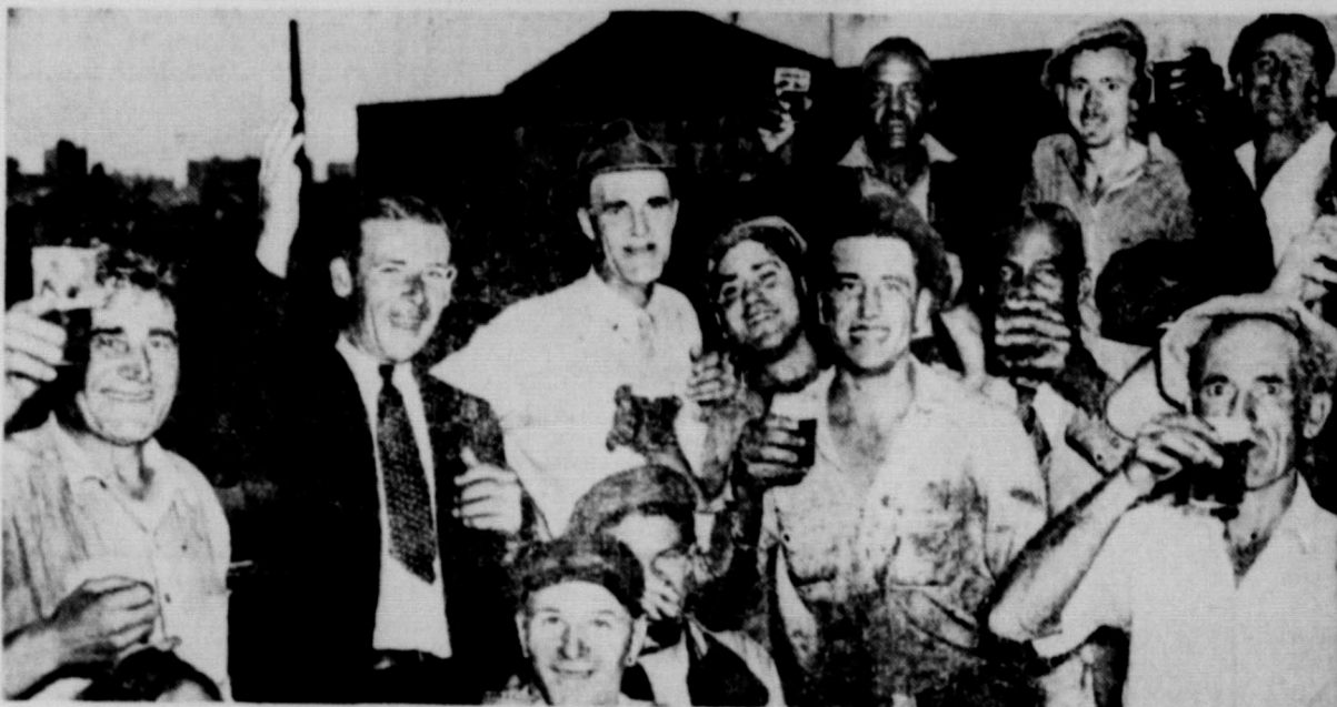
A buffet luncheon on a Forest Hills, N. Y., roof garden was the reward tendered WPA workers at the completion of a road project in that city. The luncheon was given in their honor by 125 merchants and property owners along a principal street which was widened, and was, according to the hosts, a reward for their speed and competence in getting the work done promptly, relieving traffic congestion.
