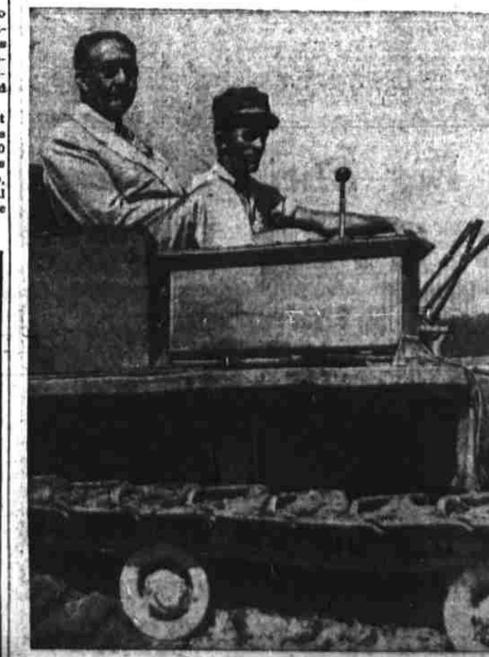
FROM GROUND UP—Rough as the ride was, Glenn L. Martin (left), airplane manufacturer, didn't mind, since the tractor in which he and a workman sat helped break ground for a huge Martin Aircraft Co. addition at Baltimore.
