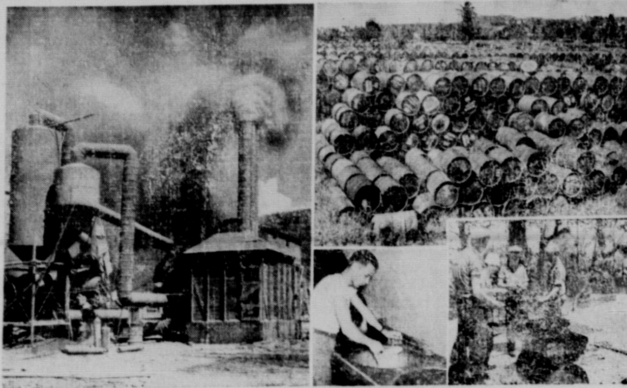
How empty oil drums are being used in the Pacific area is shown by these photos. Left, the drums were used in asphalt plant, as stacks, etc. Center, household use, wash sinks made from drums. Upper right, view of one of the oil drum farms. Lower right, used for barbecue. Other uses include bomb shelters, gateway arches, legs for water tanks, incinerators, sewer pipes and reflectors on light poles.
