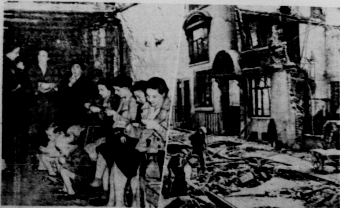
At the left is shown a "knitting bee" in a Ramsgate, England, bomb shelter. These shelters are cut through solid chalk, 60 feet below the surface, and accommodate about 50,000 persons. The women are knitting comforts for the warriors. Right: Repairing watermains and light conduits in Ramsgate after a Nazi air raid.
