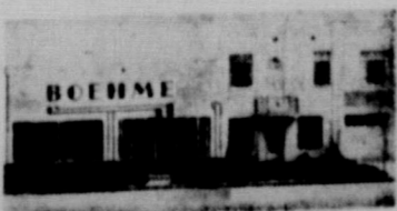
Our New Plant, Built in 1941
