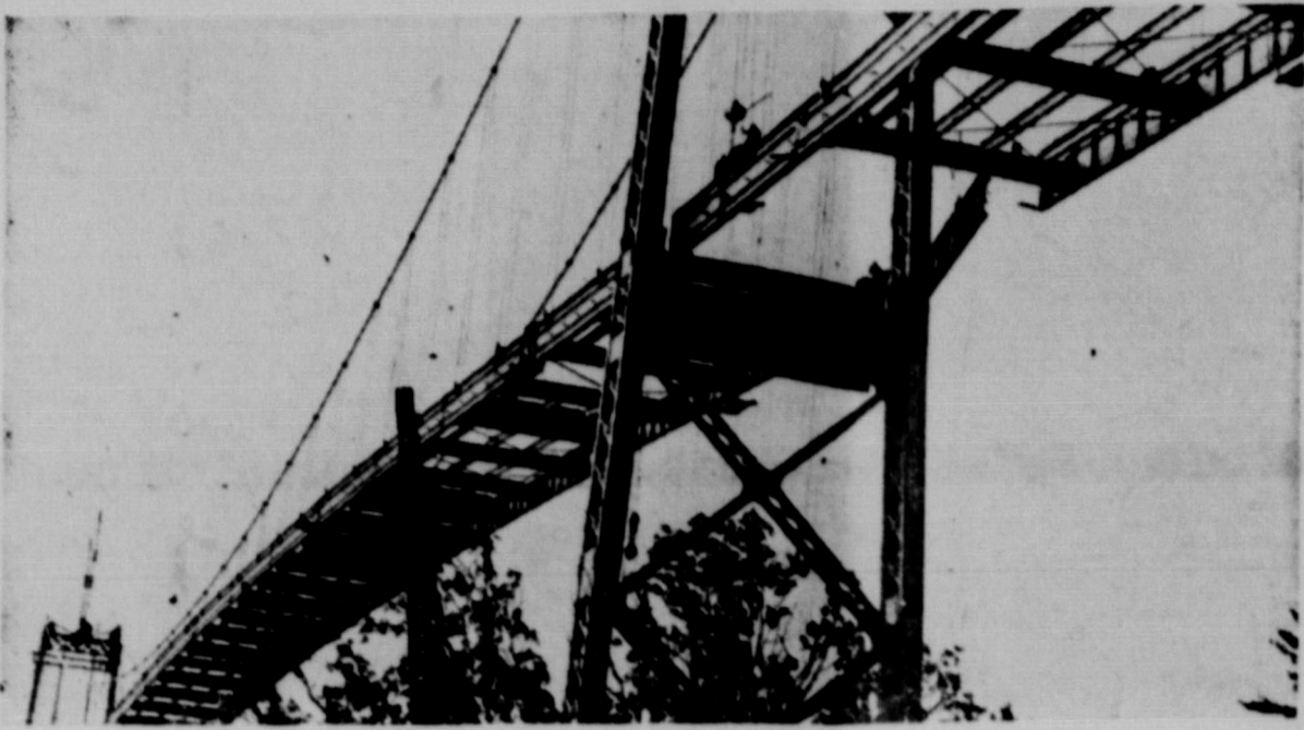
Workmen close the last span in the huge Thousand Island bridge at Alexandria bay, N. Y., which will be dedicated today in elaborate ceremonies. President Roosevelt and Prime Minister Mackenzie of Canada are among notables invited. The bridge crosses the St. Lawrence river and connects Collins Landing, N. Y., with Ivy Lea, Ont. It consists of five spans.
