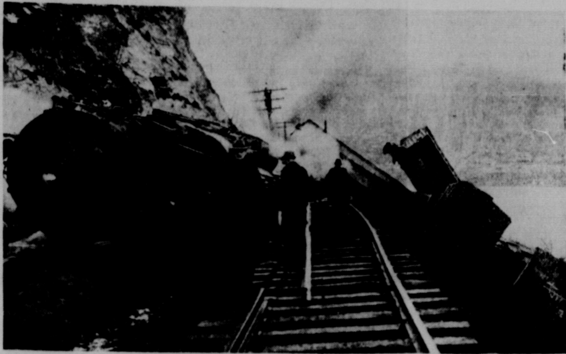
Rocks loosened by recent storms slid to the railroad tracks three miles north of Easton, Pa., causing this locomotive and 12 cars to crash down the embankment to the water's edge. Two of the cars were actually upended in the swollen Delaware river. The engineer and fireman were taken to a hospital.
