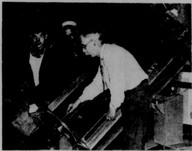
Dr. Charles Greeley Abbott, secretary of the Smithsonian institution and director of the American Astrophysical observatory at Washington, D. C., is shown setting up his solar boiler at the Great Lakes exposition at Cleveland. The device, hailed as science's first successful effort to translate solar energy into usable power, would yield a total of 70,000 horsepower on cloudless days, according to Dr. Abbott.
