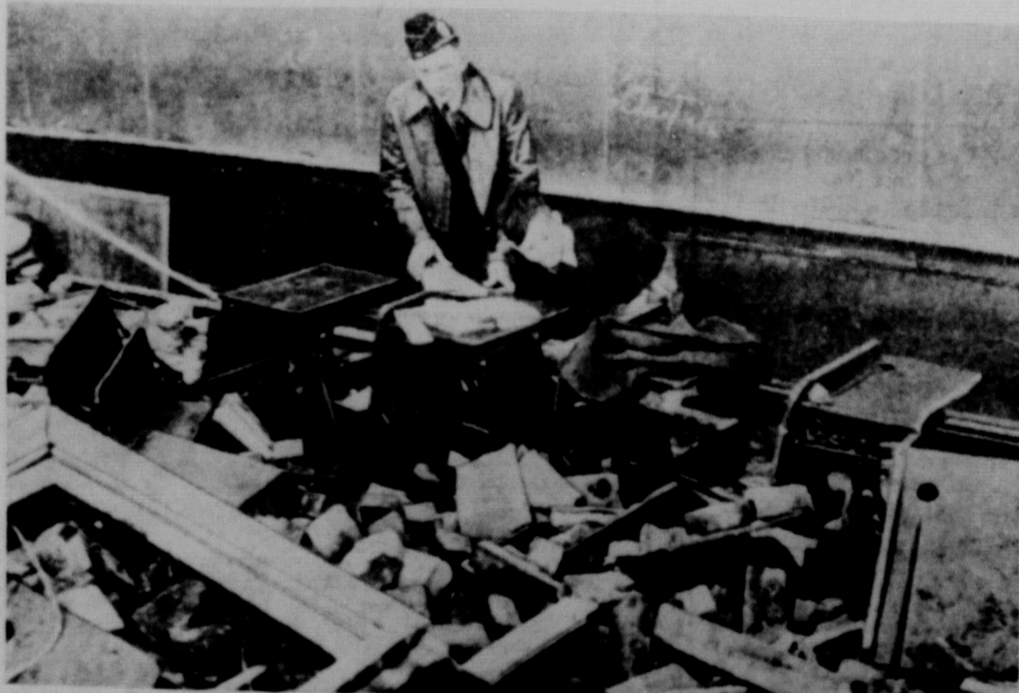
A tornado which swept destruction from Arkansas to Illinois wrecked this school at Columbus, Kan. Luckily none of the pupils were in their rooms when the twister hit. This picture shows a member of the American Legion with his little son as they recovered his things from a desk in the wrecked school room.
