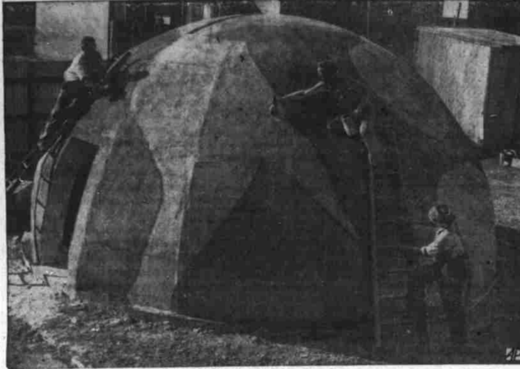
'DOME OF SAFETY' DOWN UNDER. —Constructed of 66 tons of concrete, this "dome of safety" built for protection against possible air raids in Sydney, N.S.W., comfortably seated 60 persons. Victor G. Steer, architect at Sydney Technical College, developed the shelter, using this design as affording greatest strength with use of least material.
