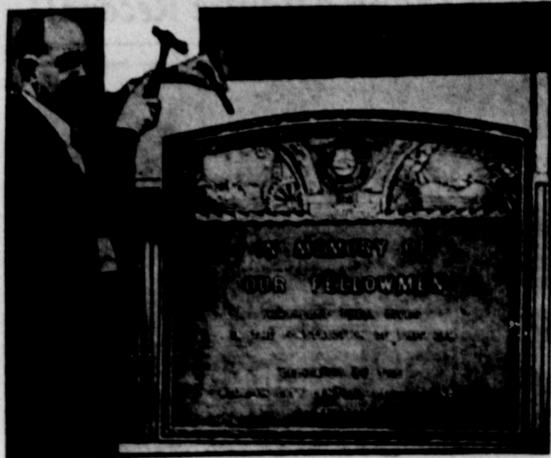
Wiley Rabun putting the finishing touches to the bronze plaque which has been set in the Nevada canyon wall near Boulder dam as a memorial for the men who have lost their lives in the construction of that great project.
