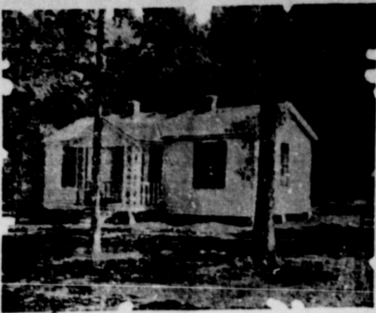
One of the model homes built in Mississippi county, Arkansas, in a project for which $1,500,000 of government funds was allotted and a tract of 16,000 acres of cut-over land bought at $2.50 an acre. The houses have been built at an average cost of $1,100 each.
