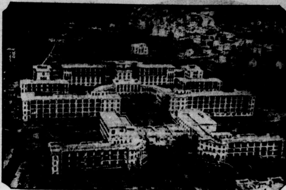
An aerial view of the huge building project now nearing completion in a Rome suburb and which will be the "Benito Mussolini Institute" for the fight against tuberculosis—probably the biggest institution of its kind in the world. The building will contain 1,391 beds and will specialize in tuberculosis in women and children. The best physicians in Italy will be members of the hospital's staff.
