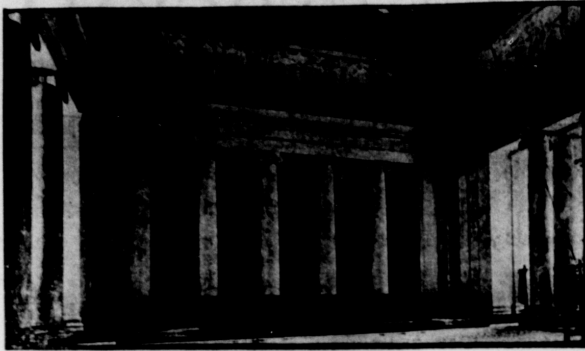
This is the almost completed chamber for the United States Supreme court in the new building which the highest tribunal will occupy in the fall.
