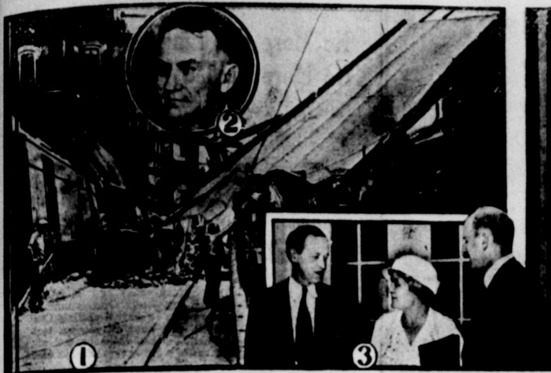
1—A Washash railway train ran berserk, leaped a siding and struck a support of this bridge in St. Charles, Mo., causing it to collapse. Two men passengers of an automobile carried away with the bridge were injured, as was a woman when her car tore through the wall of her hotel nearby. 2—John Monroe Johnson, of Marion, S. C., assumes his duties as assistant secretary of commerce, succeeding Ewing Y. Mitchell who was ousted and wrote the President that "graft and corruption" abounded in the department. 3—Harry L. Hopkins (left), works progress administrator, and Ewing Y. Mitchell, secretary of the treasury, leaving White House with Josephine Roche, assistant secretary, after discussing new National Youth administration which she will head.
