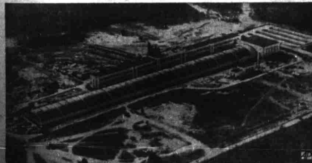
INSIDE THIS TUNNEL—SHIPS will be tested, as to design and serviceability, at the new U. S. model basin at Carderock, Md. The 1,500-foot "tunnel" shelters two basins, one shallow and one reaching a depth of 22 feet. This is an official U. S. navy photo.
