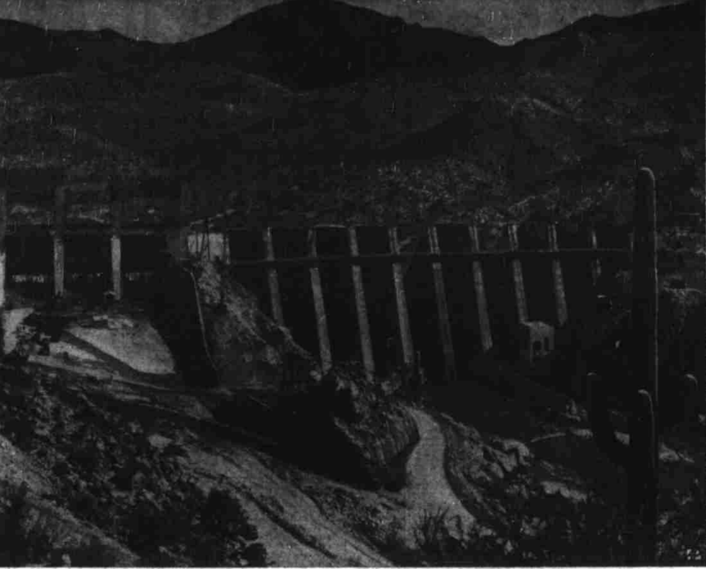
FRAMED BY THE ARID DESERT for which it is being built, the Bartlett dam on the Verde river in Arizona will provide a supplemental irrigation supply for the Salt River valley irrigation project. The dam, seemingly lower than the cactus on the right, is actually to be 270 feet high—the highest of its type in the world. Multiple arches will permit the piling-up of 200,000 acre-feet of water in a great reservoir from which water supply can be taken as needed. The dam is being constructed by the U. S. Bureau of Reclamation.
