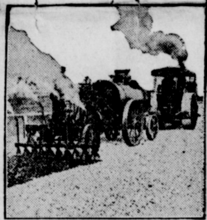
Building a Good Road in Massachusetts.
