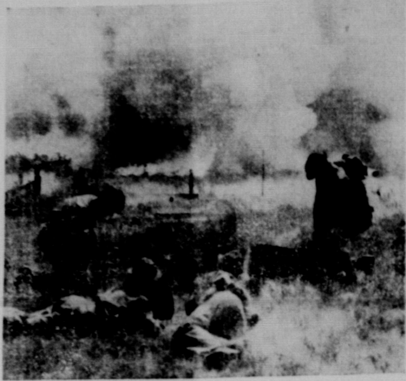
A barrage of 25 shells is fired from "Livens projectors" during the army's chemical warfare demonstration at Edgewood arsenal, Maryland. The projectors are used to throw destructive chemicals against the enemy, or smoke bombs to screen troop movements. Men in the foreground are telephone operators in contact with advance forces and the "plunger" man who sets off the charge.
