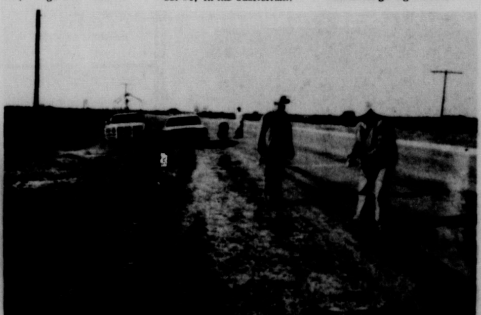
GETTING READY FOR SMOKEY IN THE SKY -- If you are wondering about the strange markings in the highway, we can give you some information. DPS personnel and Highway Department employees spent several days last week marking every 800 feet along Hwy. 290 and I-10. The purpose of the markings are to enable the DPS helicopter clock and catch speeders. Vehicles will be clocked from the air and speeders will be stopped and ticketed, by Highway patrolmen on the ground. There will be no more warnings by Co'ses.
