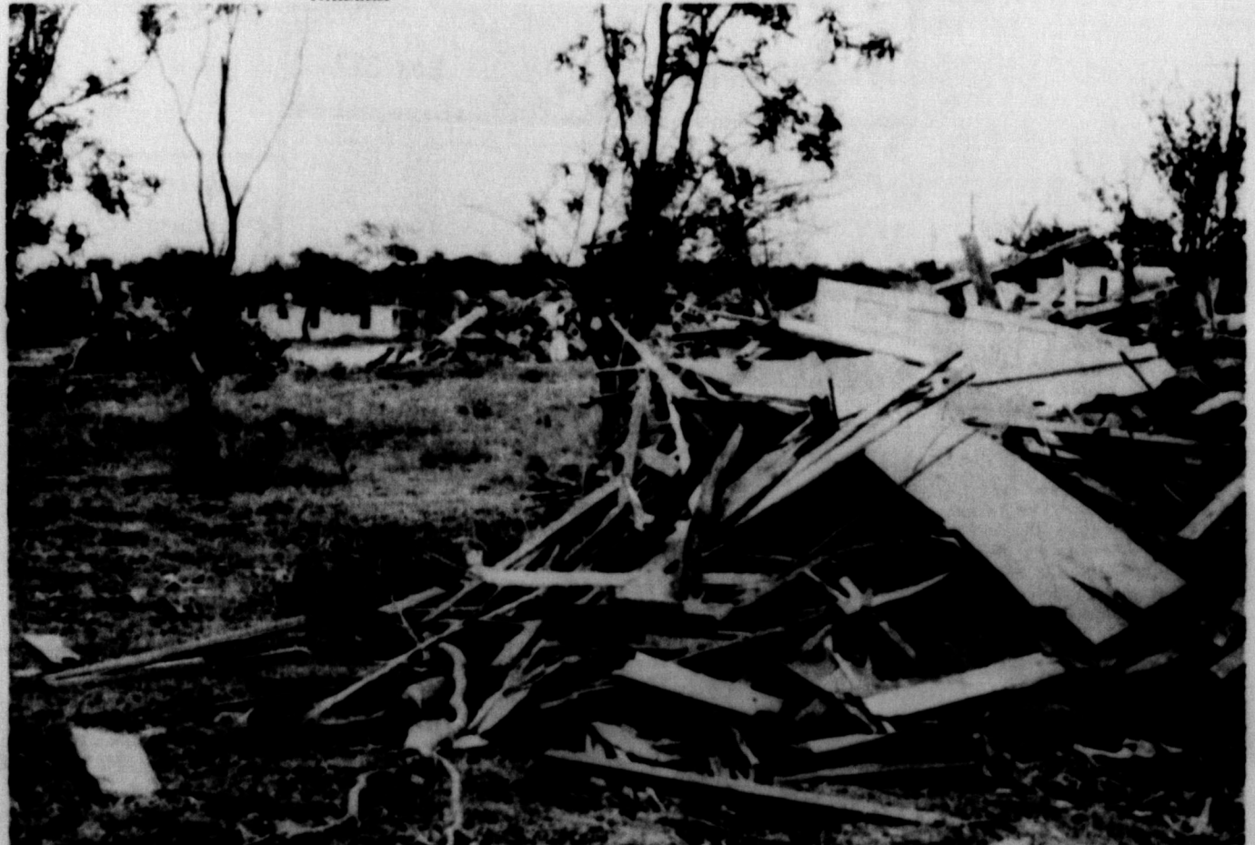
CLEARING THE PATH FOR INTERSTATE 10 through Ozona, piles of rubble stand where houses were located south of town near 14th St. The Mt. Zion Baptist Church may be seen in the background still standing. However, the heavy equipment at the rear seems to be saying "you're next." The church building will
