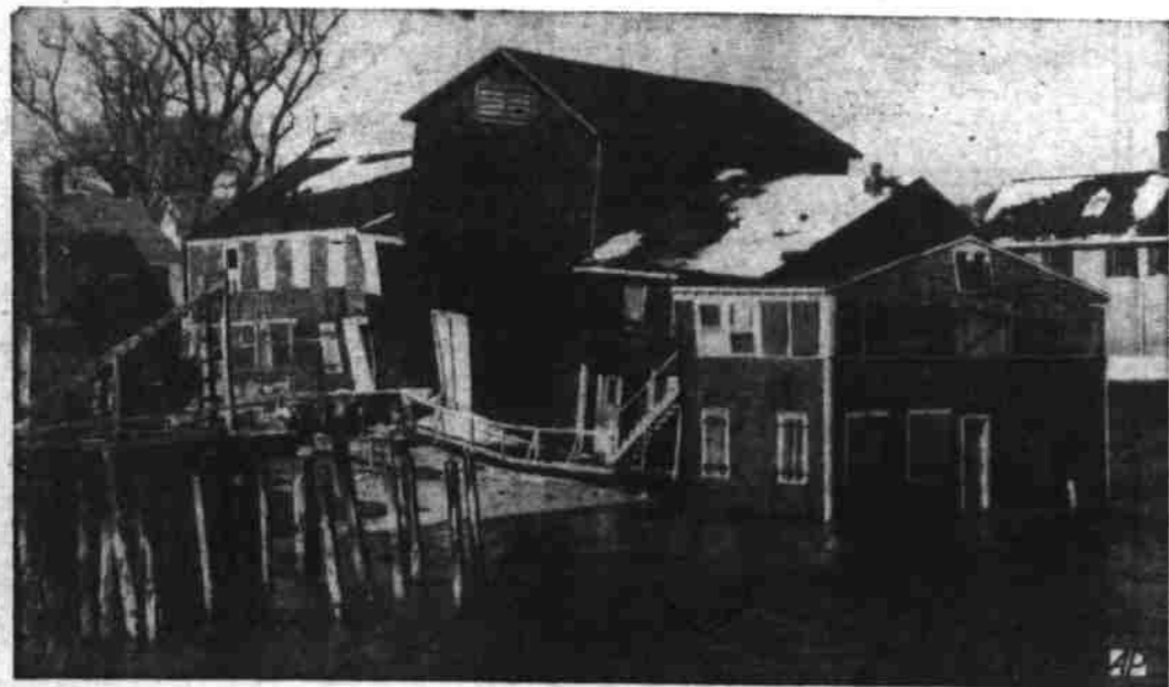
NATURE WRITES AN ENDING —Ice-filled seas so battered supports of above historic Wharf theater at Provincetown, Mass., that it slid into waves. It's oldest summer theater in U. S.
