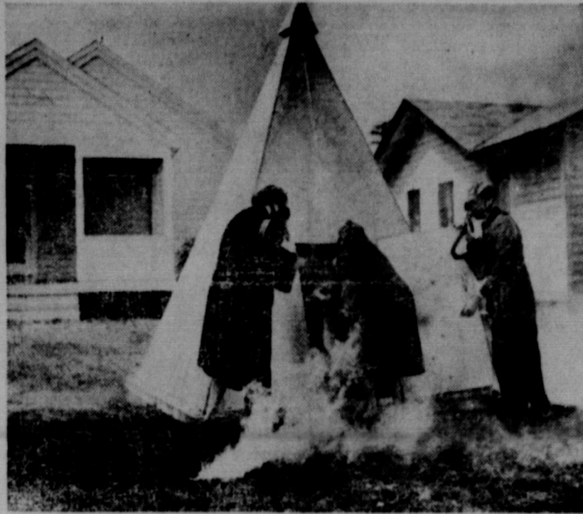
Mass production air raid shelter, shown during a tryout in Boston. It is bolted on a concrete base. Ventilation comes in at the top where the little cone crowns the steel pyramid. Yes, this shelter can accommodate 12 people. With air raid alerts on both coasts, interest in shelters is increasing. Some can be bought for as little as $200.
