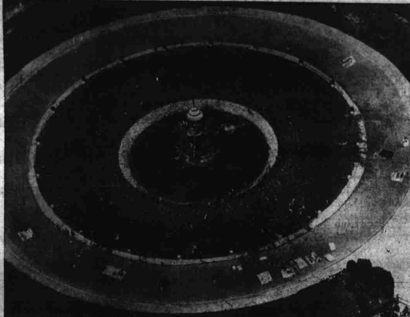
SERVES 1,798 IN TOWN OF 7,000 —Seashore Pool, in Lebanon, Ind., (population 7,000) can accommodate 1,798 persons daily. Center is 18 feet deep, with shallow water next, sloping up from 4 1/2 feet to a sand beach and greensward.
