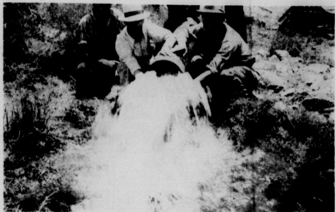
AMPLE WATER FOR OZONA USERS—Water from the 450 foot well atop water works hill, recently drilled, was flowing at the rate of between 450 and 500 gallons per minute when the above picture was taken Sunday morning. The well was given a four-hour test Sunday, pumping between 450 and 500 gallons a minute, and the water was not lowered in the hole. Another well is being started at once, the two to be equipped with centrifugal pumps and present small wells abandoned.
