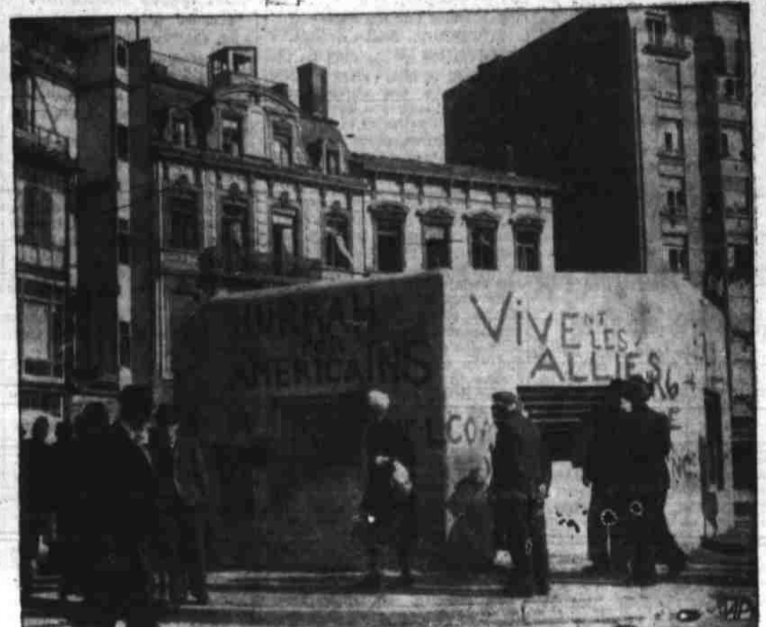
SIGNS ON LIEGE PILLBOX —A German pillbox in the heart of Liege, Belgium, bears new signs of welcome to the Allies painted by residents of the city.
