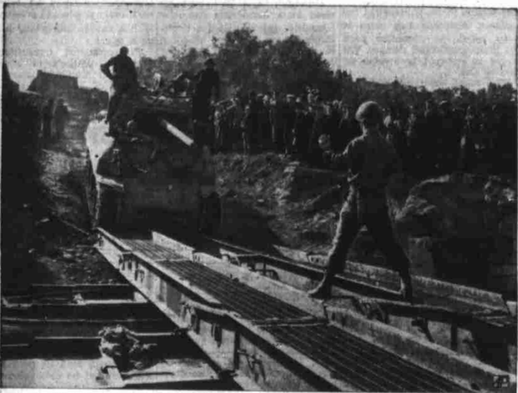
U. S. TANK CROSSES MEUSE —A U. S. engineer guides a tank driver onto the treadways of a bridge built across the Meuse River in Belgium to aid the Yank advance.
