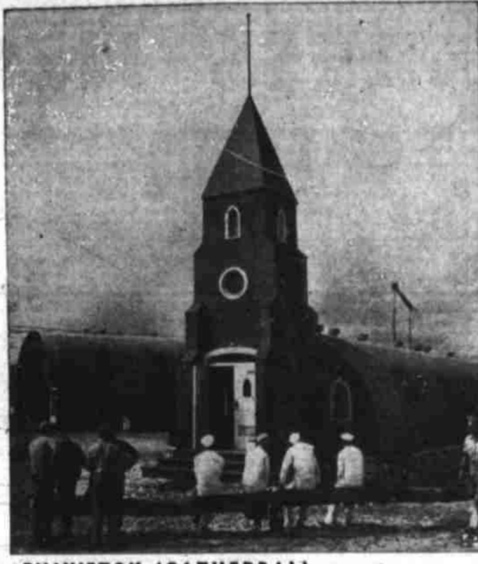
ENIWETOK 'CATHEDRAL'—Navy officers and enlisted men wait for services to start in this church on Eniwetok in the Marshall Islands group, made from a Quonset hut by adding a formal entrance and a conventional steeple.
