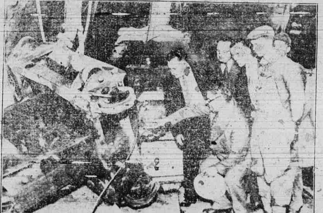
Three workmen were killed and six others injured in Chicago when a cable broke and a bucket elevator plunged 185 feet to the bottom of a water tunnel. Officials and workmen are shown examining the elevator after the accident. (Associated Press Photo)
